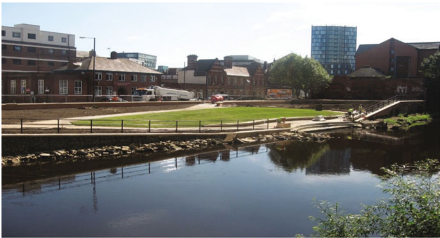
Fig. 2 Flood defenses integrated with riverside parkland on the River Don in Sheffield. (Photo provided by Sheffield City Council)
