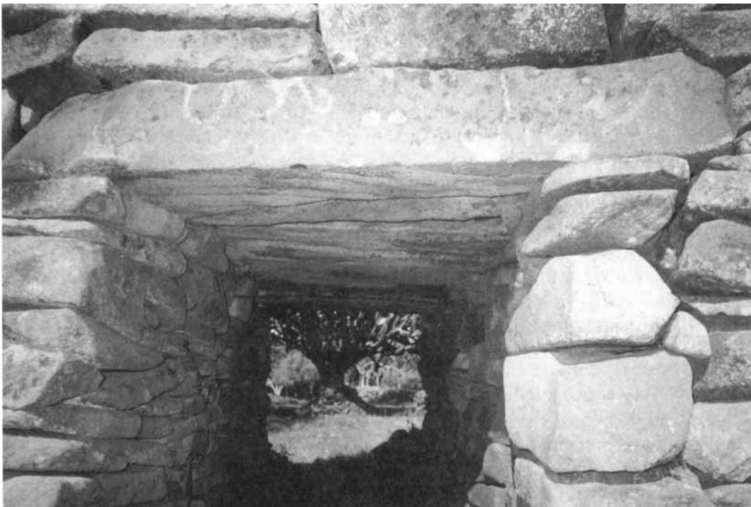
Fig. 4. An example of entrances to the Ohingni showing selected rocks of almost uniform shape.
