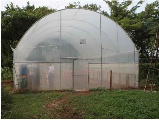
Roofing is made of polythene material while the sides is made of insect net.
