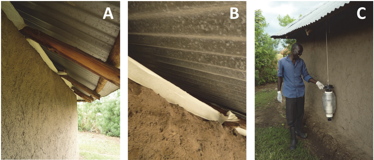
Fig 7. The components of the push-pull system. Panels A and B: The 10 cm wide strip of fabric as it was applied inside the eave, around the full circumference of the house. Panel C: The attractant baited MM-X trap as it was installed outside the house.
