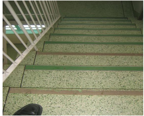
Photograph 4. 27: In-appropriate Use of Stairs to Works House. as a Design Deficiency. The stairs anti-slip has been ripped off through movement of goods which could have ferried through a goods lift.
