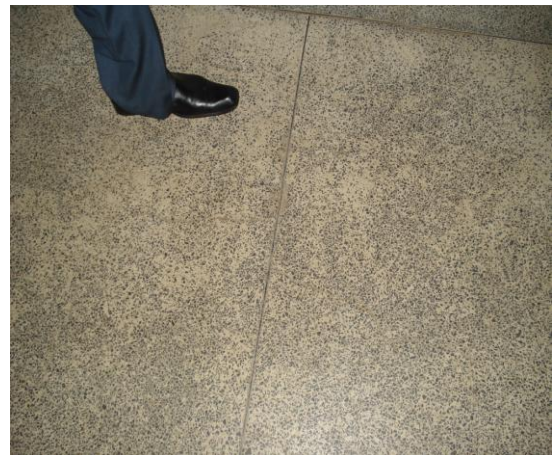
Photograph 4. 41: Quality Terrazo Floor Finish to Works House. Terrazzo is durable as well as not too costly and can withstand wetness and heavy traffic. Cost in use is very low but less appealing compared to tiles.
