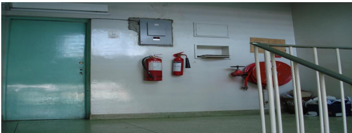
Photograph A14: Power Consumer Unit and Fighting Equipment in Magereza House.
