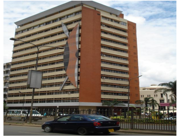
Photograph 4. 39: Painted External Façade of Protection House, a Non-cost Effective Finish. The external façade of Protection House is finished mainly in plaster/paint which requires frequent repainting and hence costly to maintain.
