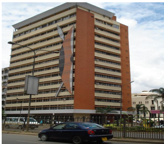
Photograph 4. 15: Recently Re- decorated and Painted External Façade of Protection House as a Major Maintenance Work.
