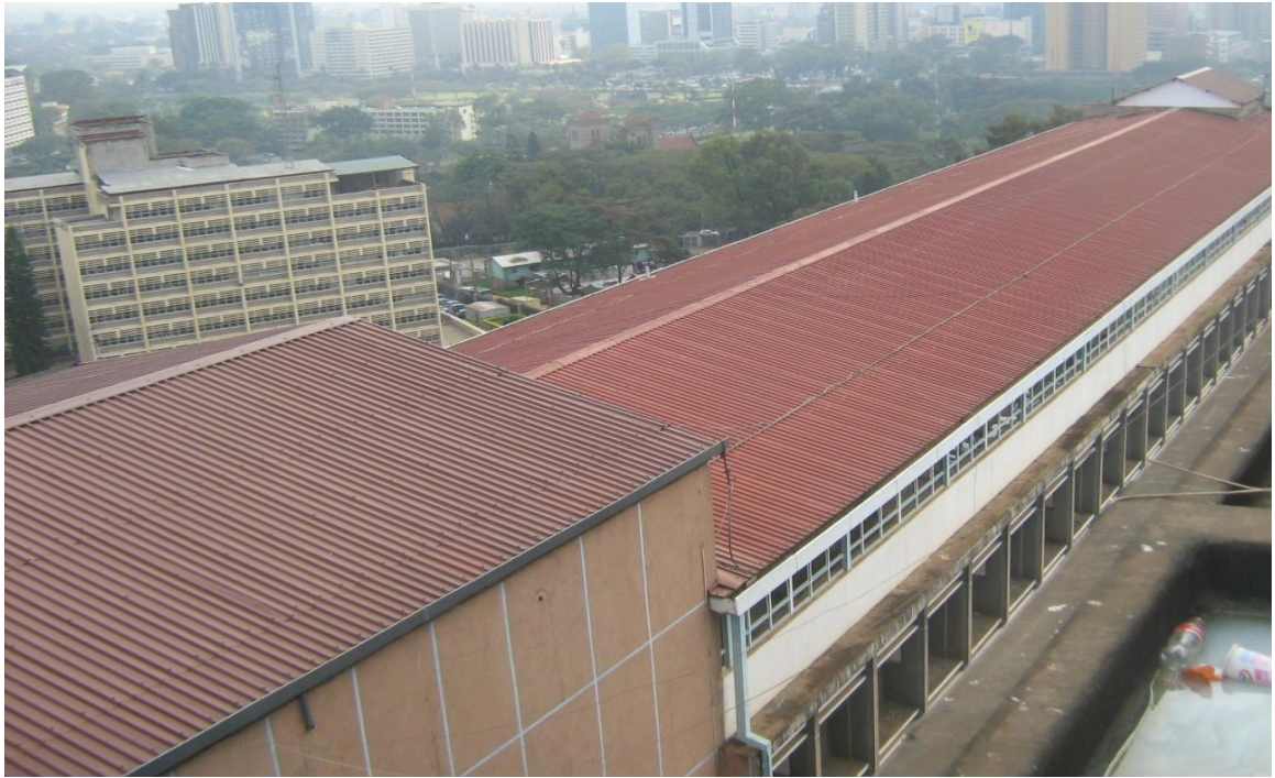
Photograph A9: Re-roofing to Transcom House
