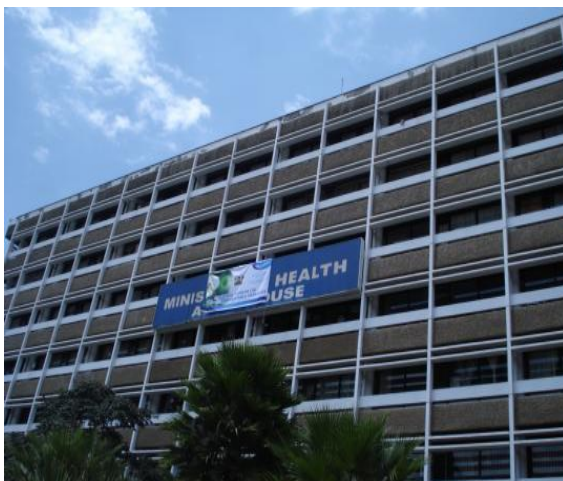
Photograph 4. 36:Fair Faced External Façade of the Afya House with Limited Painted Surfaces, a Cost Effective Finish
