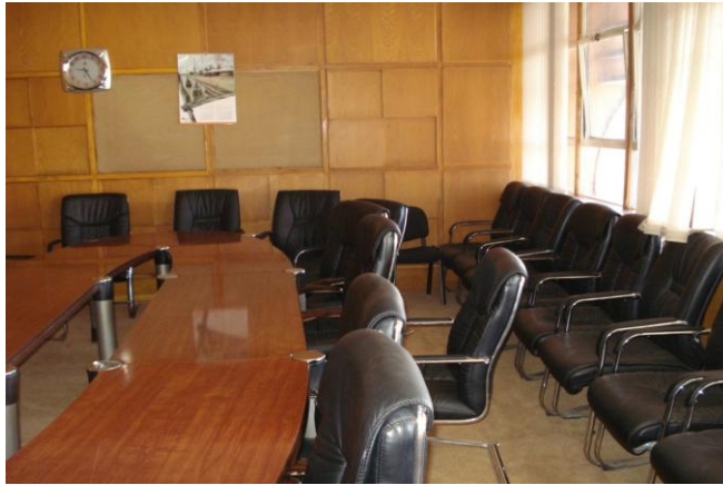
Photograph 4.34: Adoption of Timber Panels in the Chief Architect’s Boardroom, 12 th Floor, Works House, a Wall Cladding Material with Minimal Maintenance
