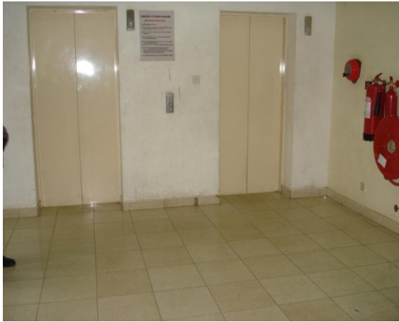
Photograph 4. 42:Quality Granito Tiles at Lift Lobby to 8th Floor, Works House. Granito tiles are more expensive than ceramic tiles but durable and can stand high impact. Cost in use is very low.
