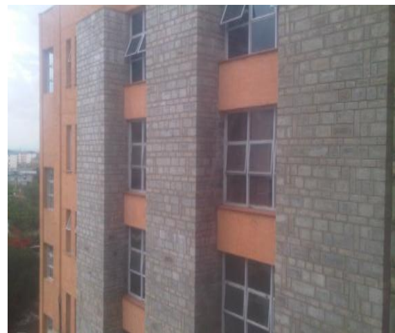
Photograph 4. 37: Keyed Masonry External Façade of Madini House with Fair Faced Beams. Madini House is mainly in keyed masonry which only requires wire brushing and cleaning at minimal cost.
