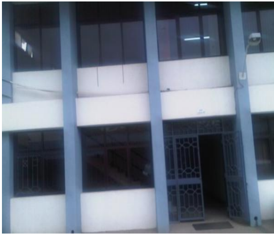
Photograph 4. 28: Painted External Facades of the National Cereals and Produce Board Headquarters, a Non-Cost Effective Finish and a Case of In-Appropriate Design.
