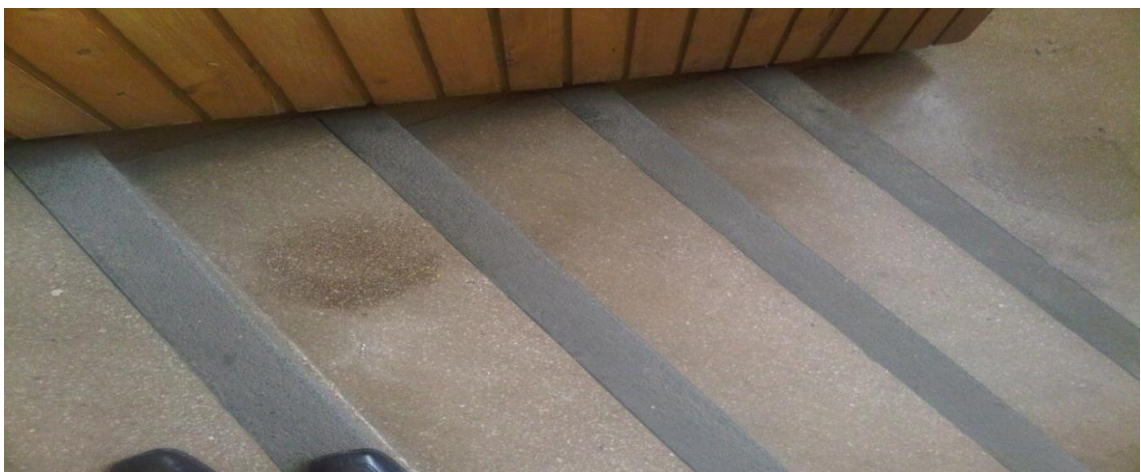
Photograph A2: Stair Finish to Safety House
