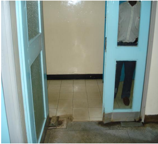
Photograph 4. 22: Re screwing of Loose Hinges to Double Door at the Magereza House as a Minor Maintenance Work.
