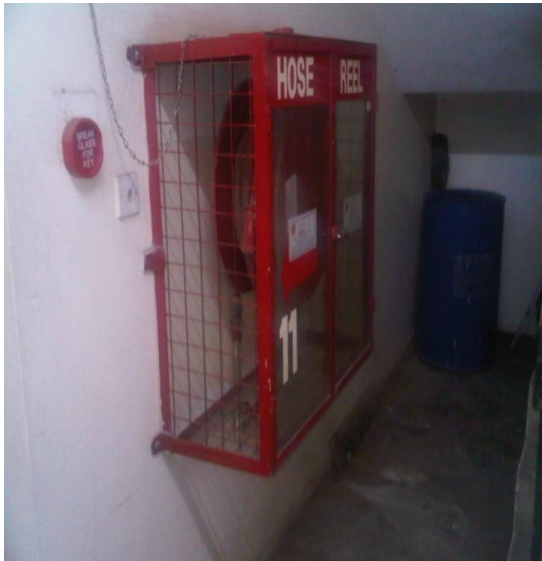
Photograph A13: Steel Caged Fire Fighting Hose Reel and Air Conditioner at National Cereals and Produce Board Building.
