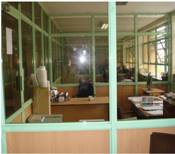
Photograph 4.32: Glass Partitions to the 7 th Floor, Works Building, a Design Concept with Minimal Maintenance Costs.
