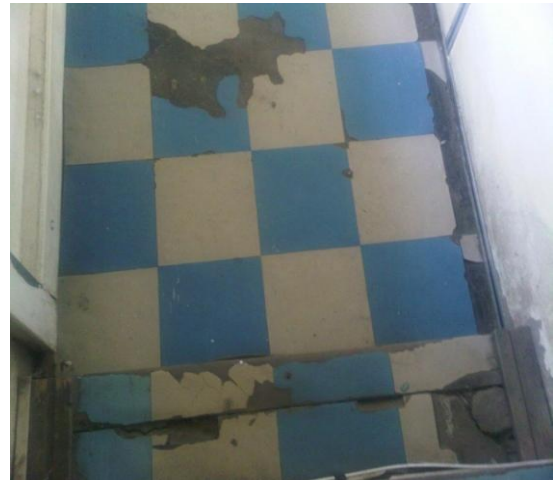
Photograph 4. 27: In-appropriate Use of Stairs to Works House. as a Design Deficiency. The stairs anti-slip has been ripped off through movement of goods which could have ferried through a goods lift.
