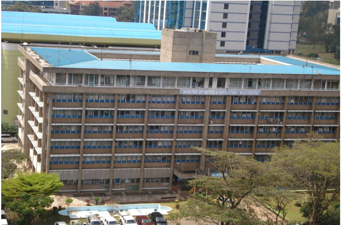
Photograph A11: Re-roofing to Maji House
