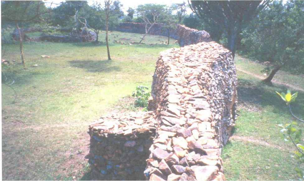
Figure 2. Thimlich Ohinga Complex site showing a section of the wall with interlocking pattern and 3-phase design used in construction for structural stability
